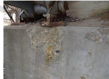
abutments and wingwalls exhibit cracks, spalls and rock pockets. Minor erosion is also present along the back face of the wingwalls, as these wingwalls are insufficient in retaining the current fill slopes due to their size and length.
