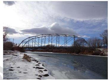
14 feet. Discussions with the MDT indicate the bridge abutments were constructed in 1946 while the truss was originally built in the early 1900's and was part of the Huntley Bridge over the Yellowstone River before being moved to its current site. Periodic maintenance and repairs have been made including replacement of object markers, installation of load posting signs and replacement of timber deck members.
