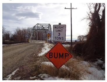
With a current useable width of 15.5 feet, the current Chance Road Bridge is too narrow to facilitate two-way travel. Carbon County has decided to utilize a 24-foot wide bridge width primarily for safe passage of two-way traffic. As the current roadway width of Chance Road is around 22 feet, a 24-foot useable width structure will accommodate future road widening along Chance Road.
