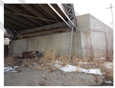
The bridge superstructure consists of a 203-foot span camelback steel through-truss. Steel stringers support the deck and transfer the load to the truss via steel floorbeams. There are
