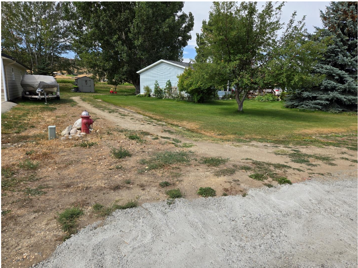
Existing Fire Hydrant on Lot 2
